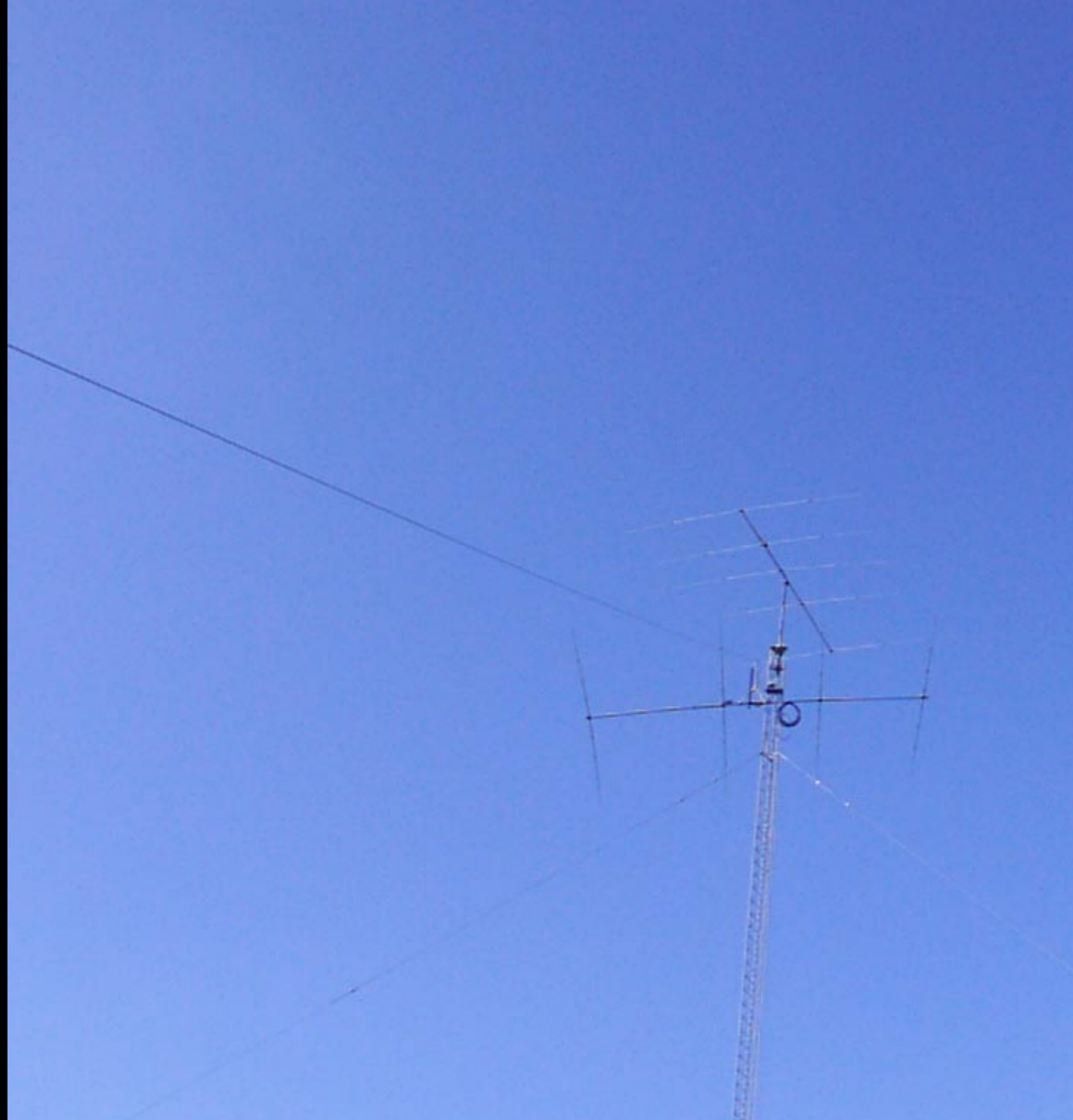
Antenna nearing the top - note how it clears top guys
